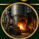
FORNO / CALDEIRA INDUSTRIAL
